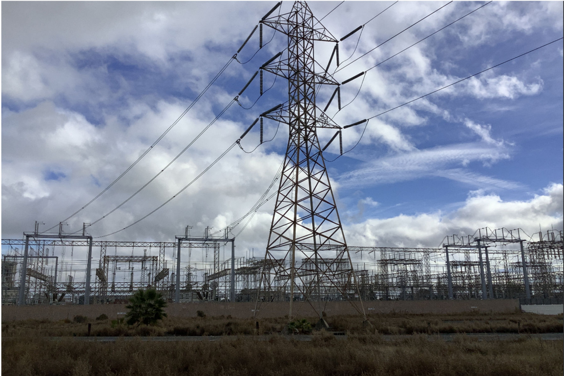
Figure 7-16. Overview of P-07-002956. View east.
