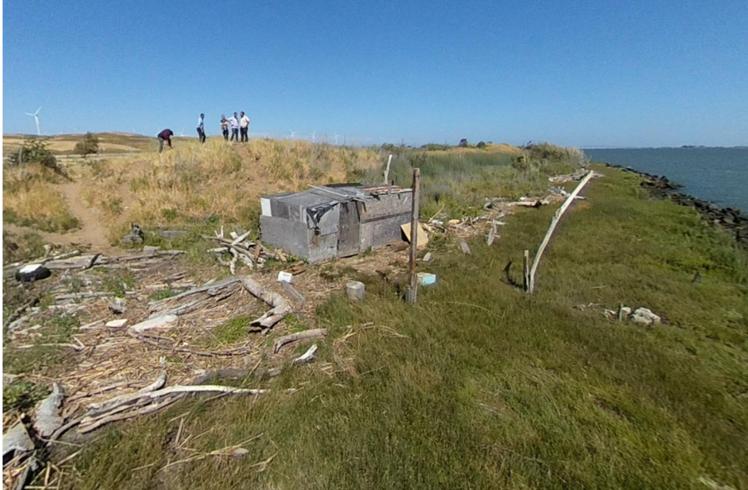
Figure 7-19. Overview of shack, facing east.
