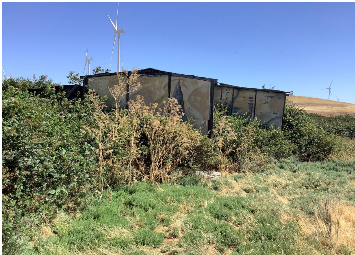
Figure 7-22. Site overview, facing northeast.
