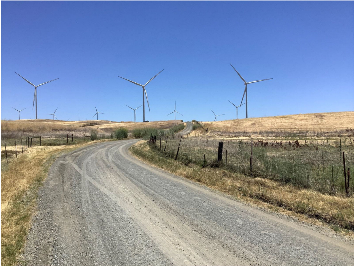
Figure 7-24. Overview of Stratton Lane, Segment 1, view east.
