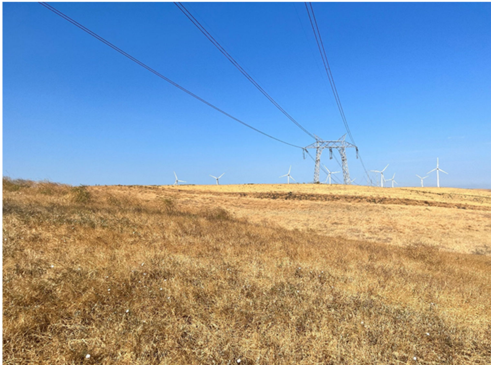
Figure 6-1 . Proposed Project overview, facing southwest.
